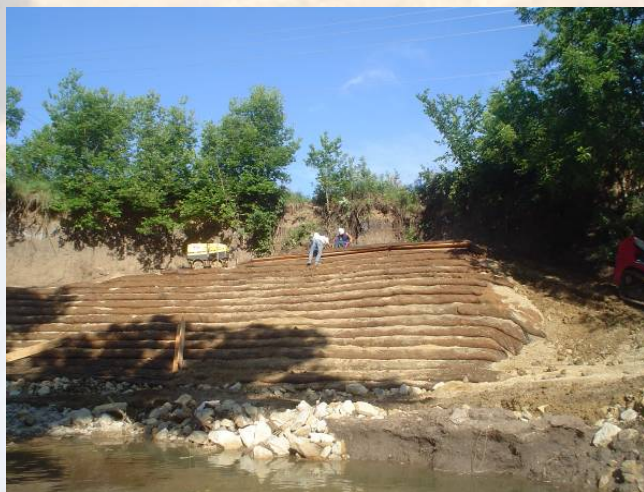
Vegetated Geo-grid – Pottawatomie Co. KS
