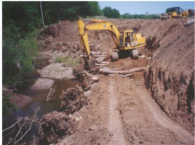
LWD – Root wad Stabilization – Sharps Creek – KS
