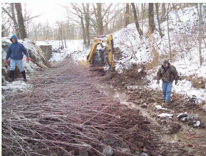
Phil Balch -Vegetated Geo-grid Installation– Wyandotte Co. KS
