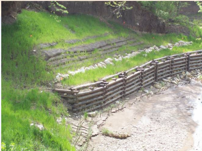
Live Cribwall – Pottawatomie Co. KS
